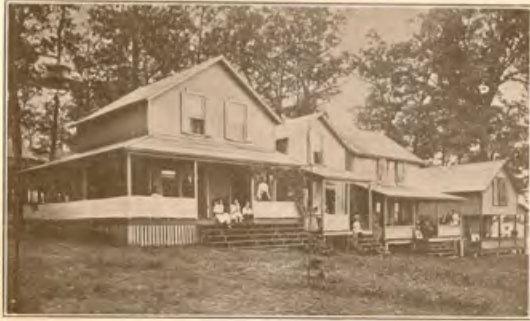
Fairview Avenue, Looking East
